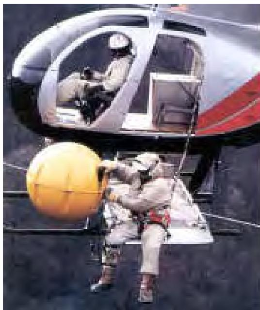
Figure 31. SpanGUARD Installation [29]
