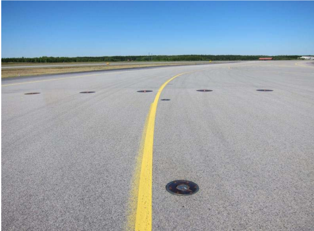
Fig. 5 Taxi line that the pilots followed. The row of five lamps from left to right is part of a stop bar, 29 June 2011.
