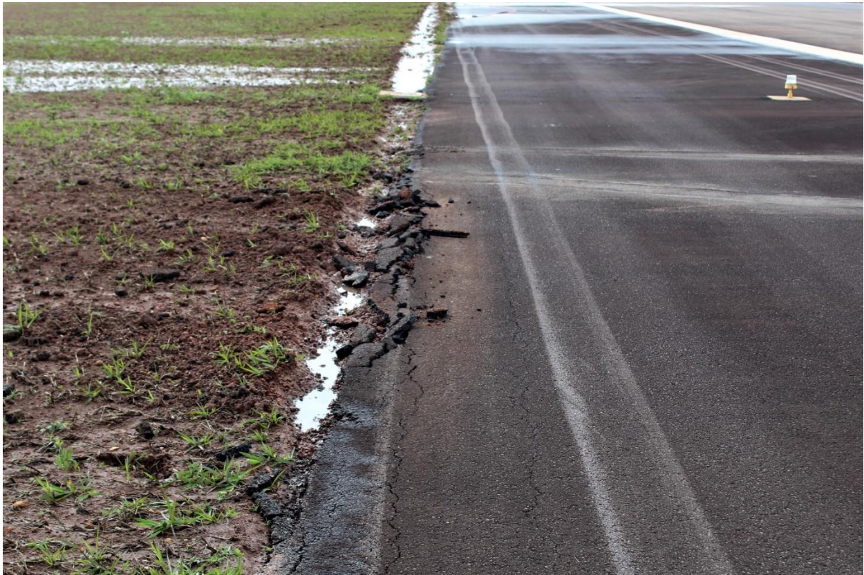
Figure 7: Damage to damage to the edge of the left runway shoulder.
