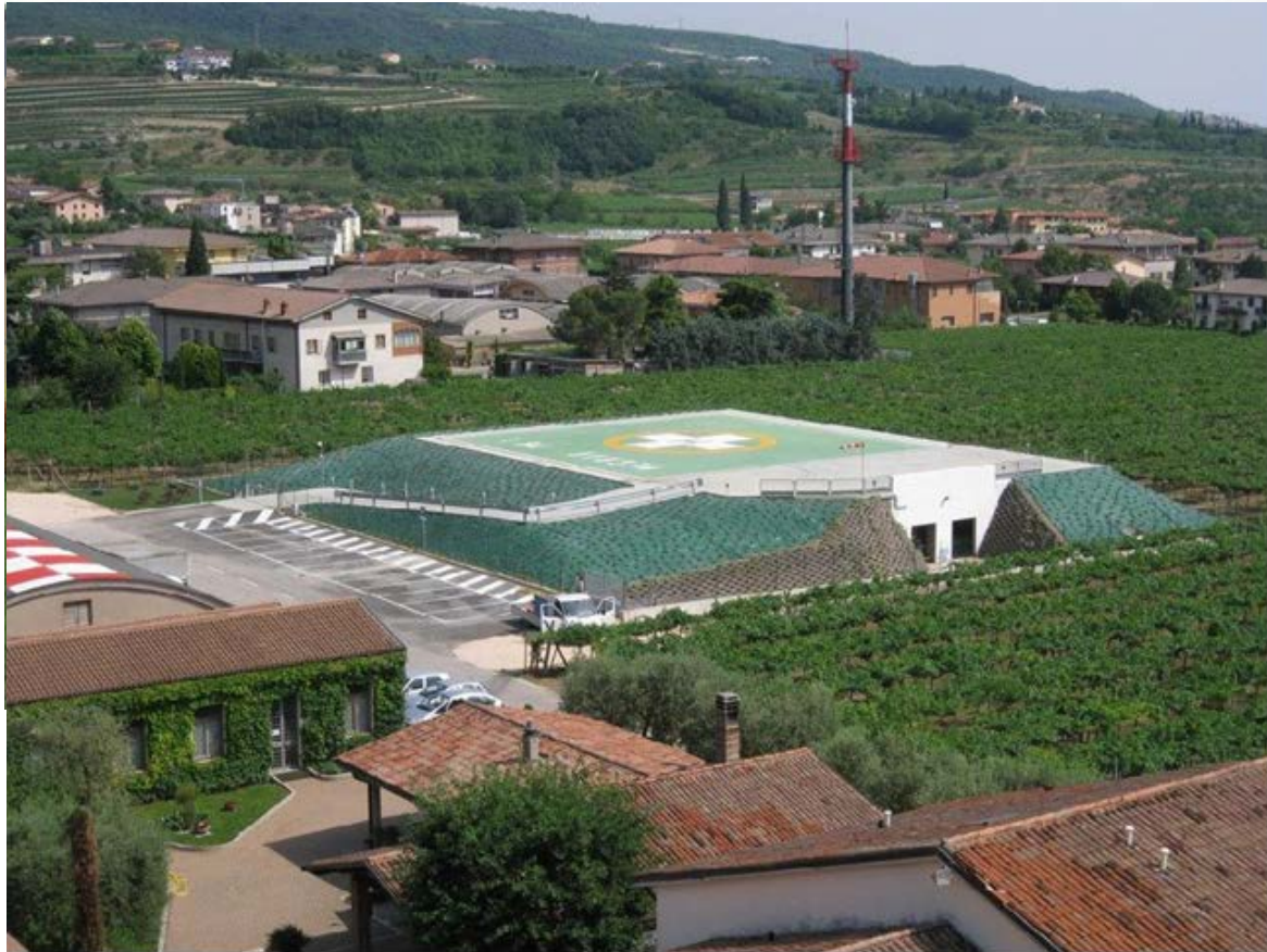
Figure 2: A mounded heliport at surface level (Ospedale Negrar)
