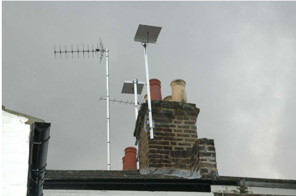
Figure 10: 1030/1090 antenna installations
