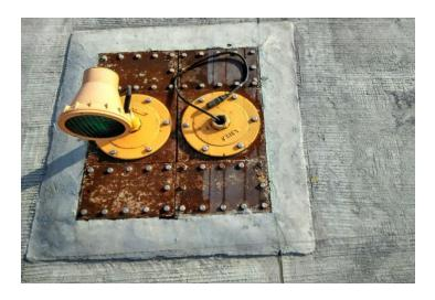
Figure A: Damage to runway lights.
